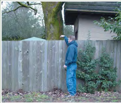
Meter is located behind the fence
