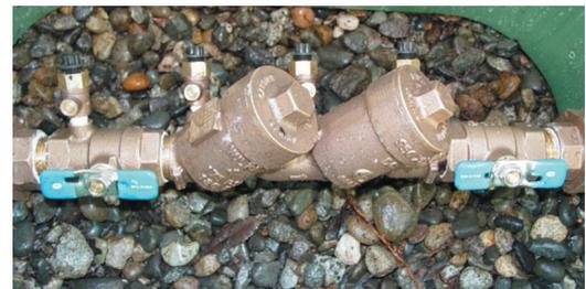
Double Check Valve Assembly used for backflow protection on irrigation systems
