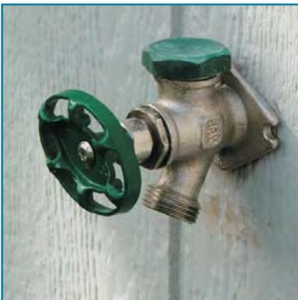
A hose bib with built in anti-siphon backflow protection.
